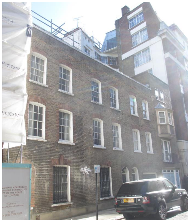
Views of the application site, Romney Street elevation
