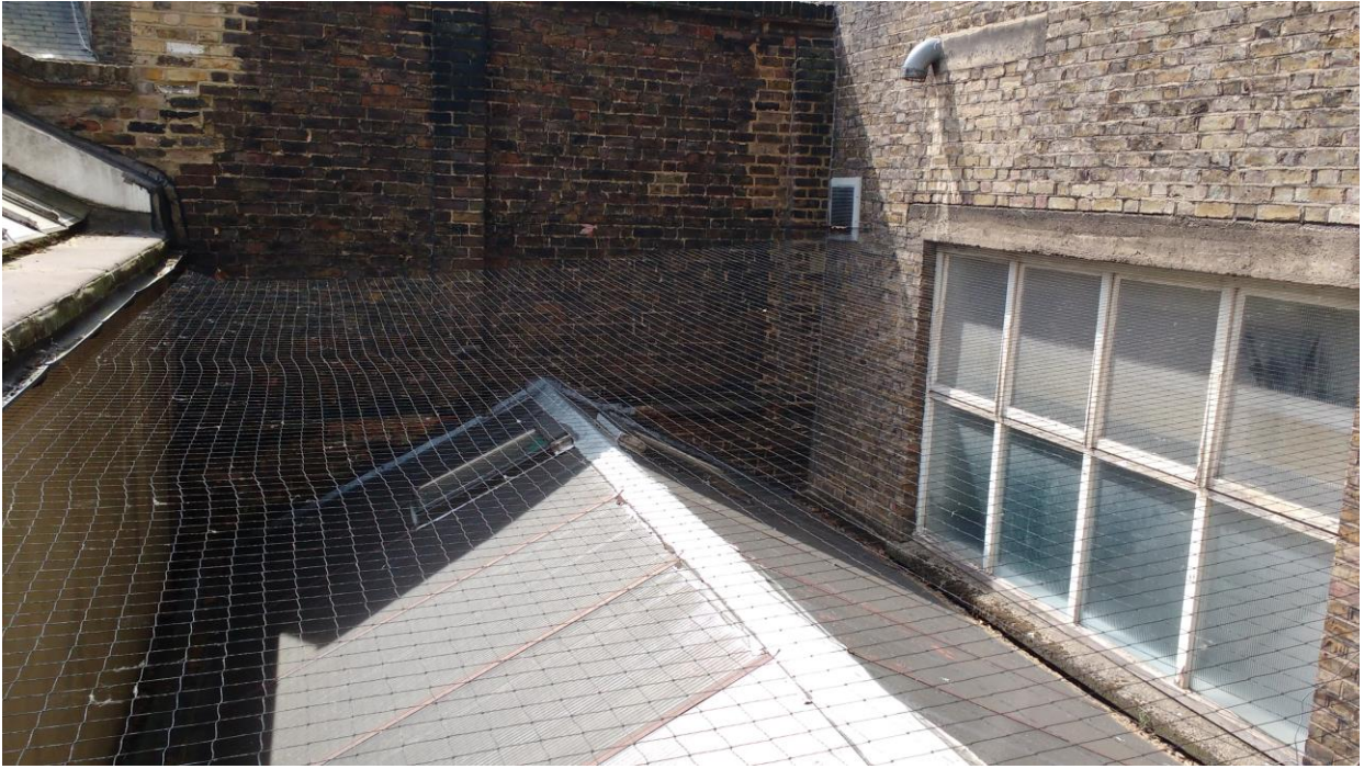
View of existing rear extension
